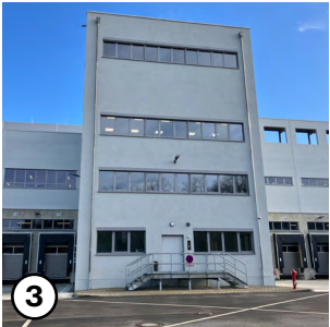
3 Registration forwarding companies/Sanitary area driver
